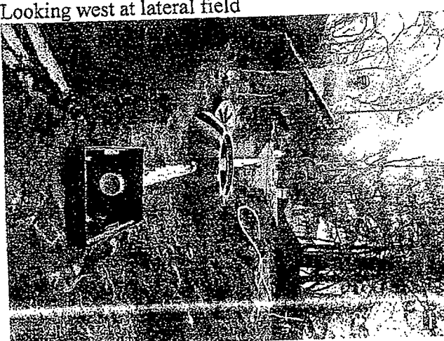
looking SE Distribution Box and tanks Tees added prior to departure
